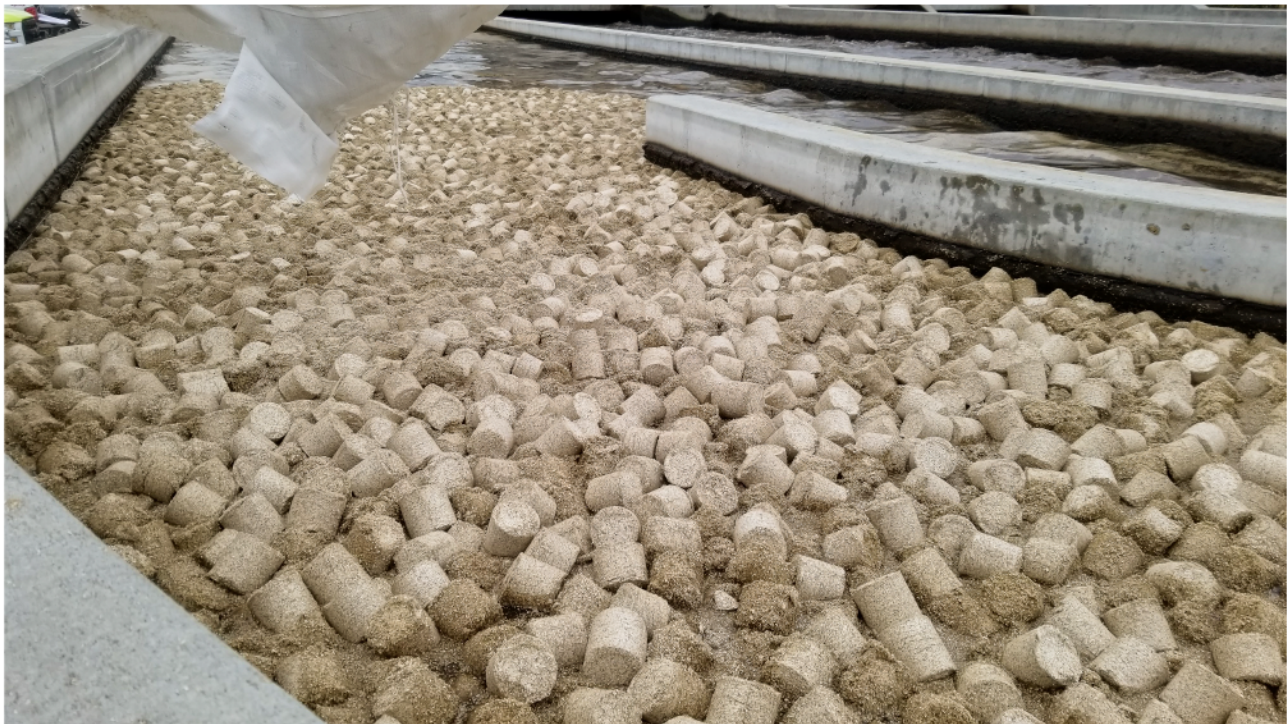
Kenaf after immediate addition into activated sludge system. The kenaf briquettes dissolve into solution.
